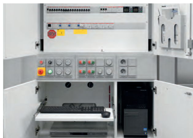
Top: electrical sub-distribution, Middle: integrated multimedia compartment
